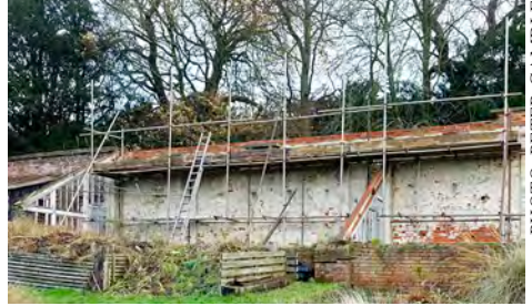
EAST WALL - RESTORATION BEGINNING
