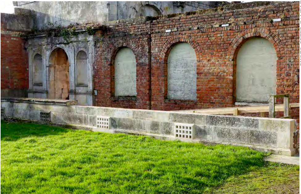
THE RESTORED LOW WALL TO THE FORMER GLAZED CORRIDOR
