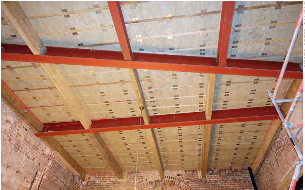
FIRE RESISTANT MATERIAL INSTALLED ABOVE DINING ROOM AT SECOND FLOOR LEVEL
